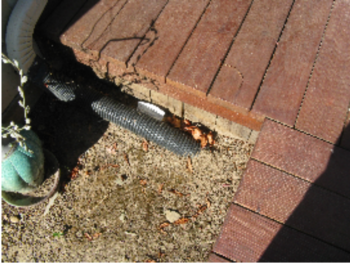
Earth/wood contact at deck
