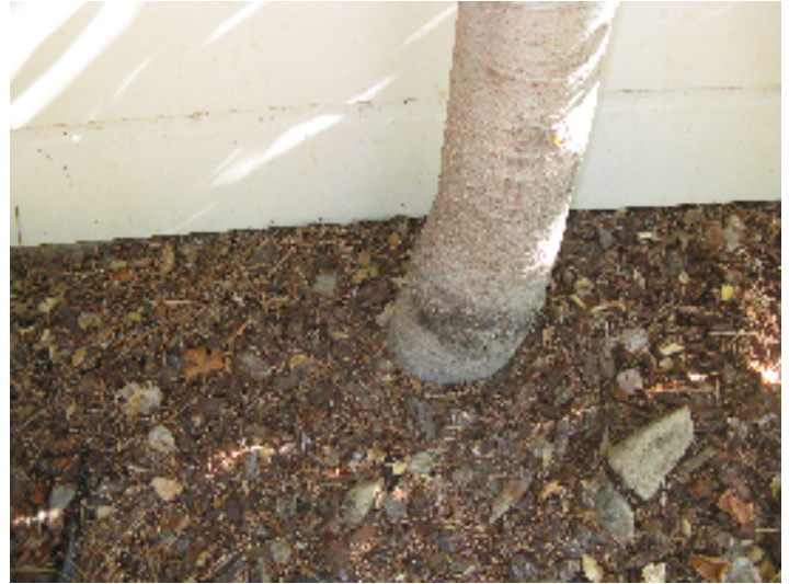
Tree too close to siding and foundation
