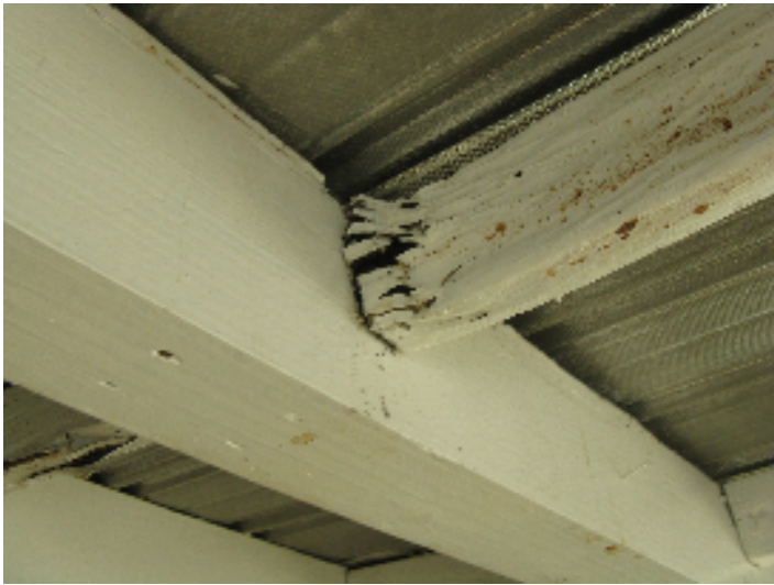
Earth/wood contact at deck
